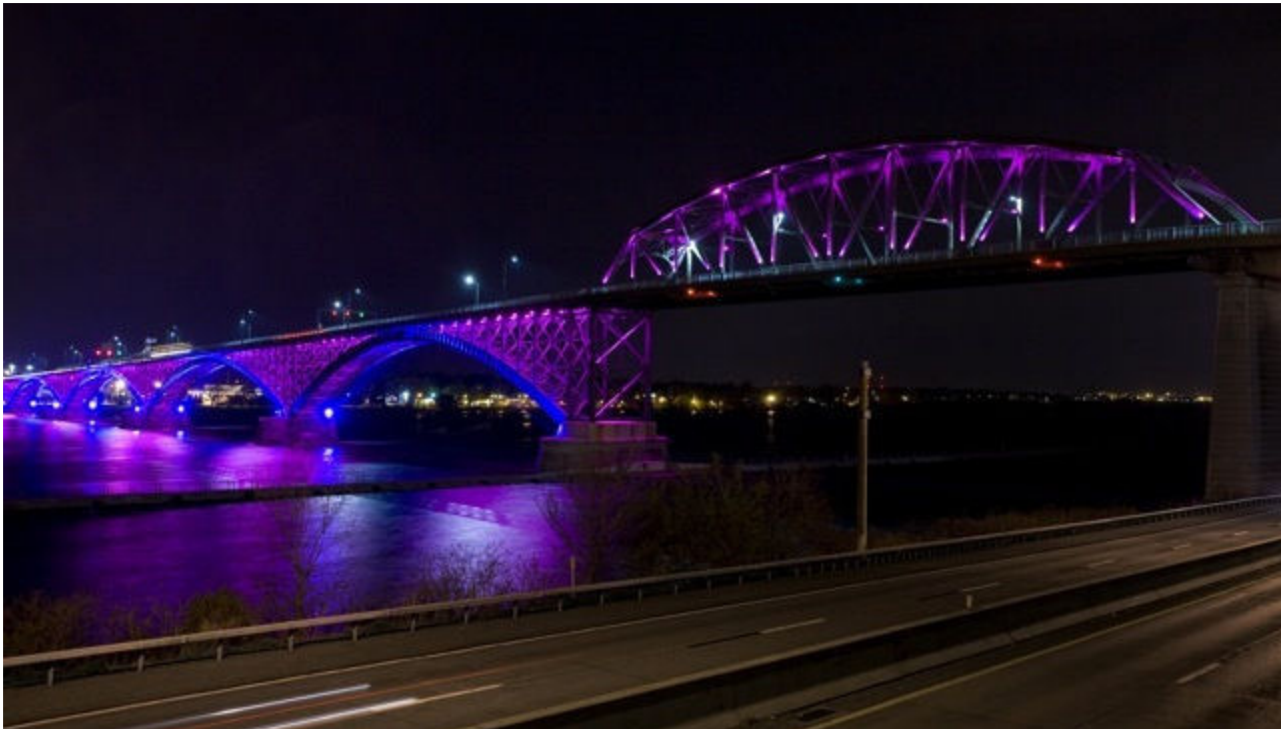
The Peace Bridge between Buffalo and Fort Erie uses some 700 RGB LED color-change lighting fixtures Philips Lighting
